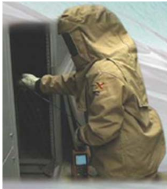
Power quality readings
