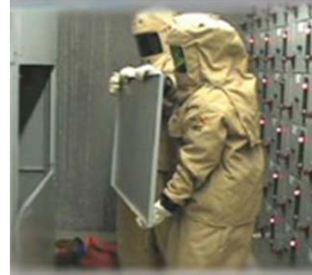
Removing fronts from high voltage panels
